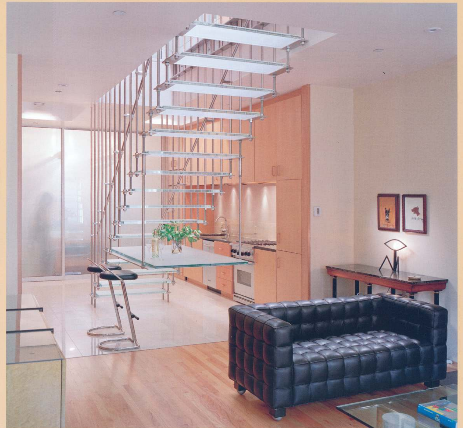
Plan diagrams (below) and an east-west longitudinal section (facing page) highlight the loft's glazed openings and the path and intensity of daylight that enters the apartment. The loft's focal point—an open-tread glass stair—allows light from a skylight above to fill the lower level and provides a unique backdrop for the kitchen eating area (above).
